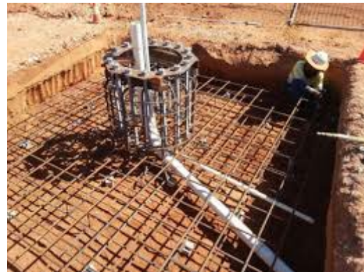
Figure 2 Pad and Pier Foundation
